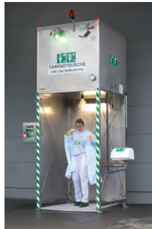
Tanknotduschen Tank safety showers
